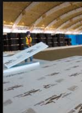
Richmond Olympic Oval STYROFOAM™ HIGHLOAD 60 Insulation is used under the ice rink to help maintain uniform, consistent ice temperatures.
